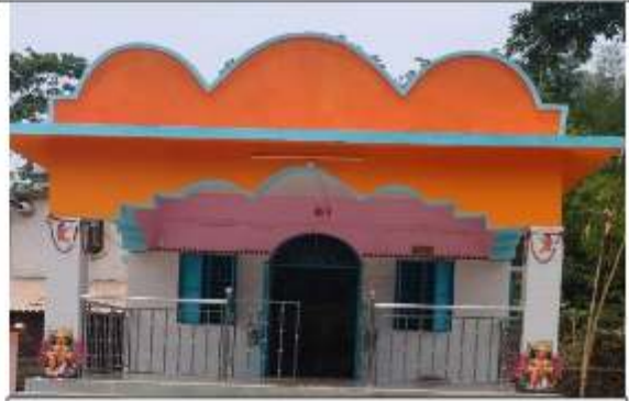
Construction of Community Prayer Centre (Mandir)
