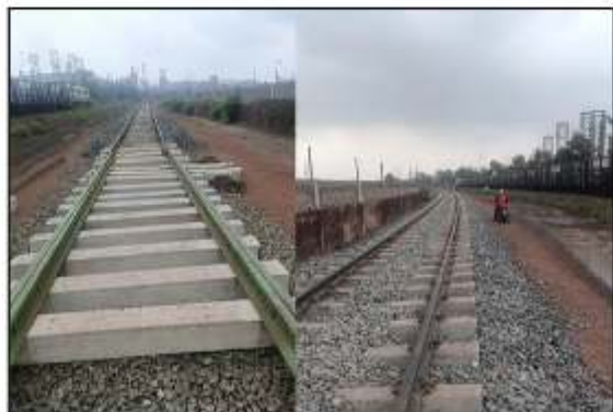
RAILWAY SIDING UNDER CONSTRUCTION
