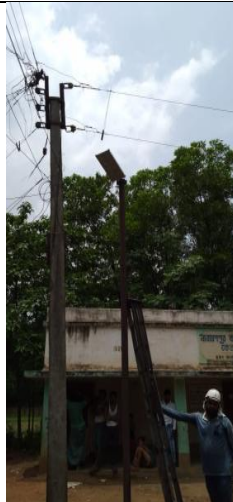
Installation of LED solar Street Lights with pole 30 nos. at a gap of 50 meter apart on road measuring 1.5 km from Charchak to Gokulpur.
