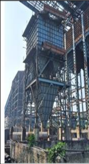
Bag filter for arresting dust emission in DRI Plant (Separation Building, Product House, Cooler Discharge)
