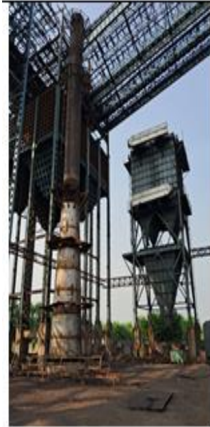
Bag filter for arresting dust emission in DRI Plant (Separation Building, Product House, Cooler Discharge)
