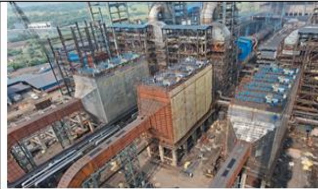
ESP for arresting dust emission in DRI Plant (2 x 350 TPD + 2 x 500 TPD)
