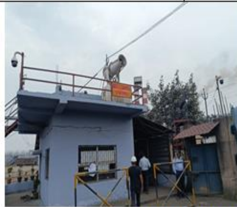
Fixed Water Mist Canon System-02 Nos.
