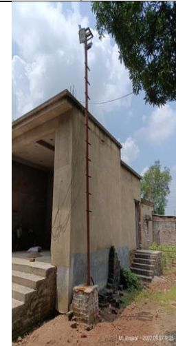
Installation of LED solar Street Lights with pole 30 nos. at a gap of 50 meter apart on road measuring 1.5 km from Charchak to Gokulpur.
