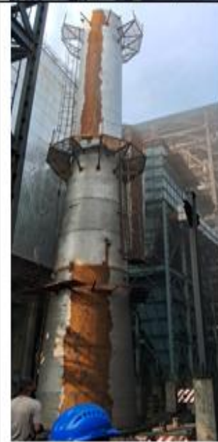
Bag filter for arresting dust emission in DRI Plant (Separation Building, Product House, Cooler Discharge)
