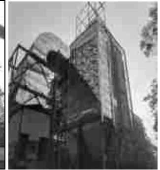
ESP of pellet plant
