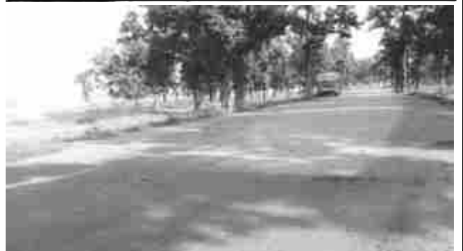
DEVELOPMENT/ REPAIRING OF ROAD
