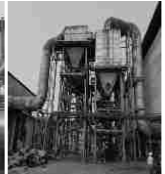
Multi cyclone sinter plant
